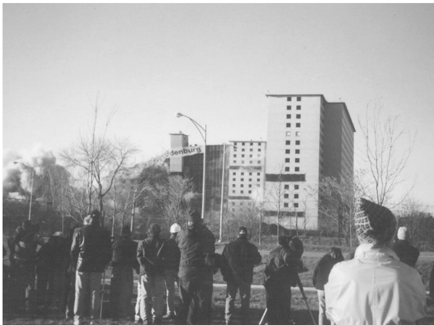
Figure 4 Spectacle of the implosion of four public housing high-rises. Author's photograph.
